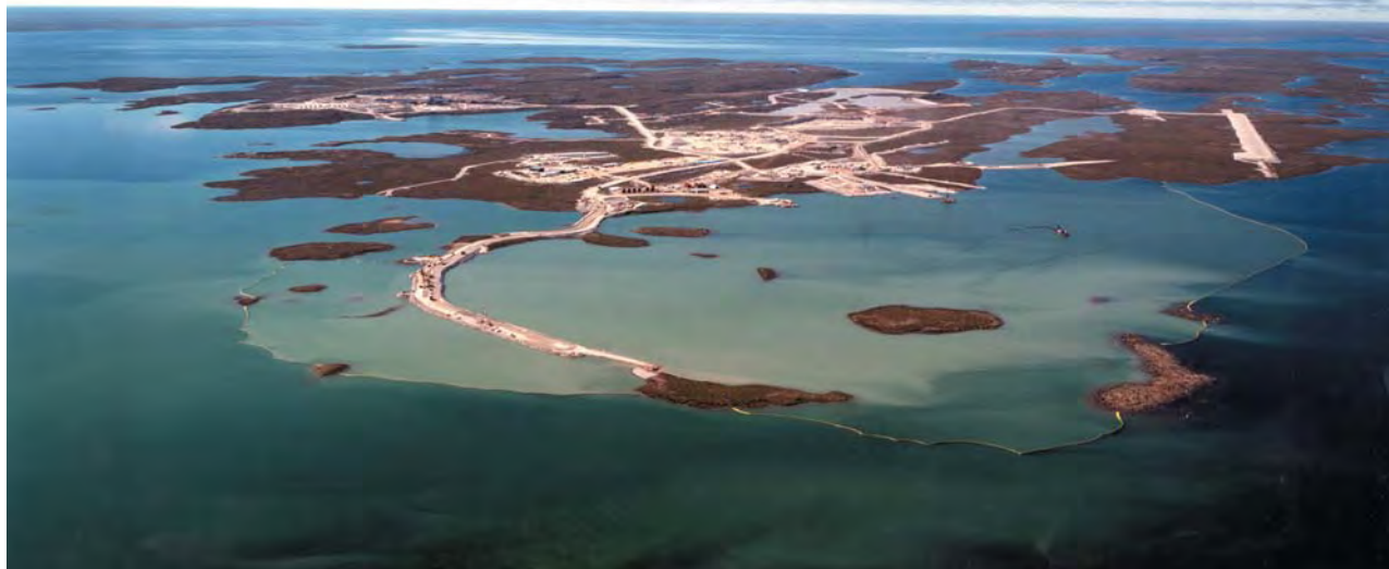
Figure 2. Construction of the Diavik mine is underway in anticipation of diamond production in early 2003. Three kimberlite pipes (A154N, A154S, and A418) are located beneath Lac de Gras in the foreground, and a fourth pipe (A21) is located under the lake on the far left of the photo. The prominent arcuate structure in the foreground is a rock dike (to be completed in fall 2001) that will be used to hold back the lake surrounding the A154N and A154S pipes to allow for open-pit mining. Silt from dike construction is carefully contained to minimize the environmental impact on the lake. The processing plant (also under construction) and camp are located in the background on the left. The disturbance in the center is a quarry that supplies rock for construction of the dike, and an airstrip is visible on the right. Photo by Jiri Hermann; courtesy of Diavik Diamond Mines Inc.
