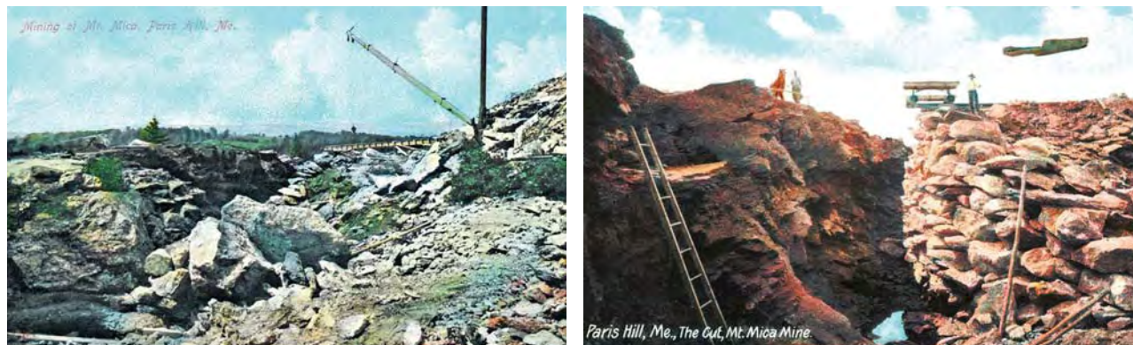
Figure 4. The images on these post cards show mining activities at Mt. Mica around the turn of the 20th century. A large derrick (left; printed by The Hugh C. Leighton Co., Portland, Maine) was used to remove boulders from a deep trench (right; printed by The Metropolitan News Co., Boston, Massachusetts). Remnants of the stacked boulders shown in the right image still can be seen today. From the private collection of Jane C. Perham.
